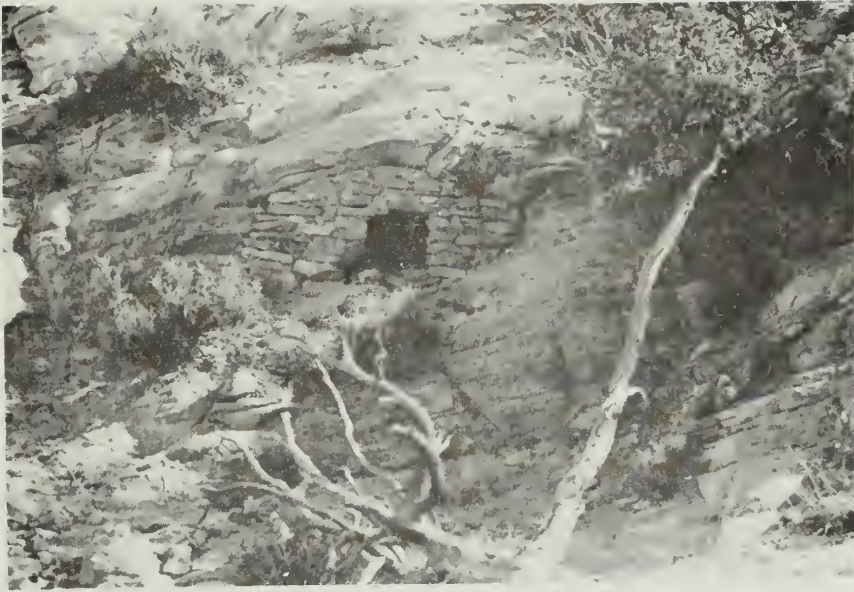
Beef Basin Planning Unit. Site 42Sa6100. Masonry wall built to create storage unit in rockshelter. Facing west northwest.
